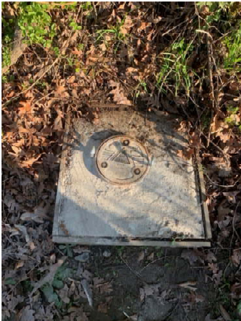
B-98 – Installed locking bar.
