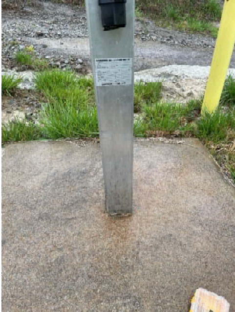
B-82 – Drilled weep hole.
