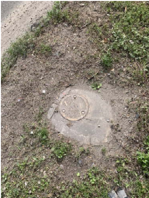
B-96 – Installed Locking bar.
