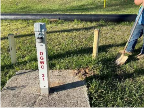
DGWC-21 – Removed ant bed.
