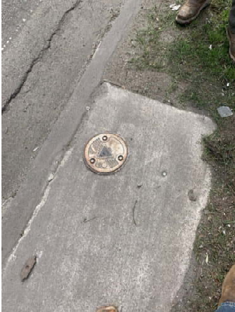
B-95 – Installed locking bar.
