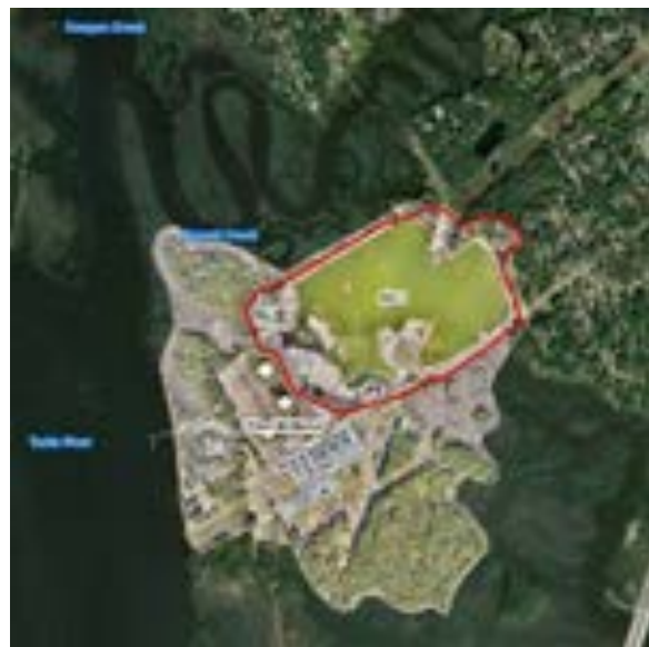
Figure 1. Former Ash Pond (AP-1) and Site.
