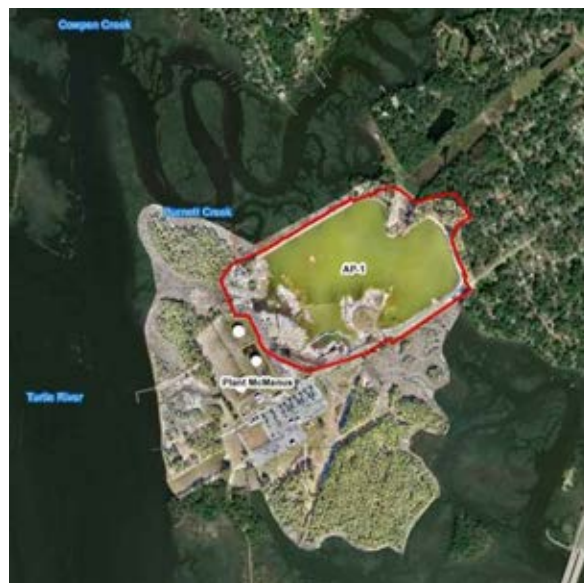
Figure 1. Former Ash Pond (AP-1) and Site.
