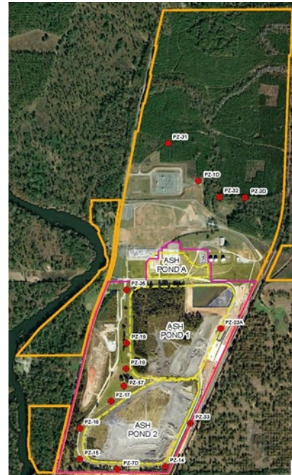
Plant Mitchell Ash Ponds A, 1, and 2
