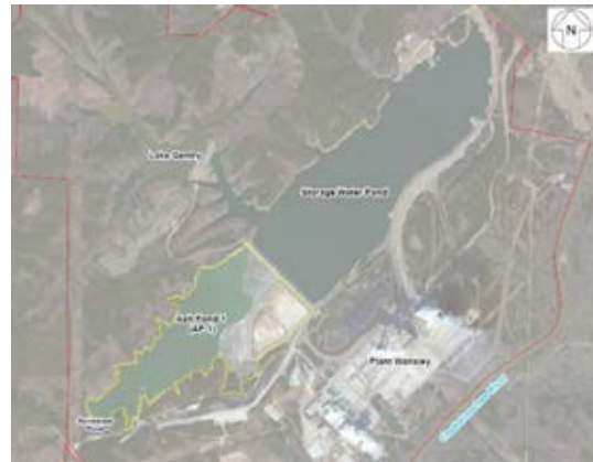
Plant Wansley and the Site
