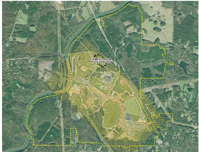
Plant Yates and the site
