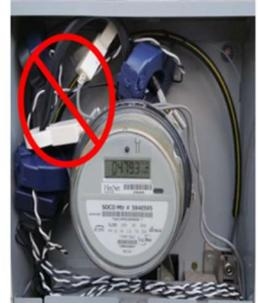
Customer owned CT meters and instrument transformers
