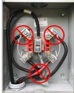
Improper routing of wires in the meter compartment, which does not allow proper clearance around the socket
