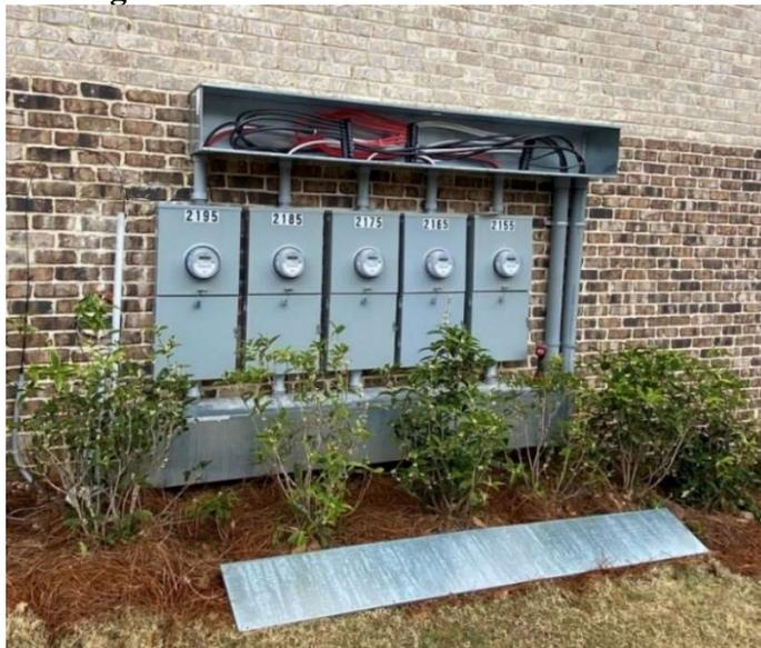
**3.3 Single Phase Meter Socket & Auxiliary Gutter Installation**
