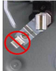
Socket lugs with factory “bypass horns”
