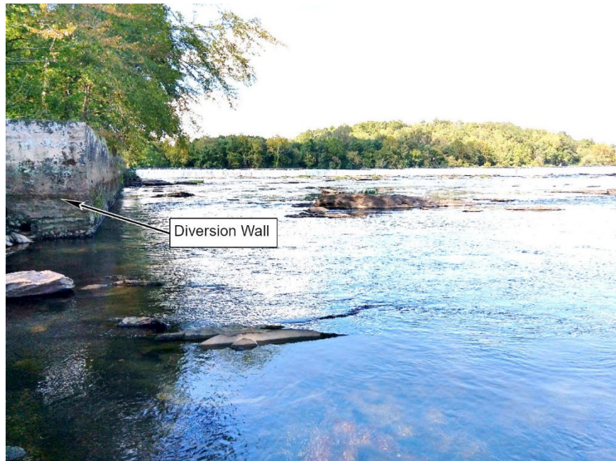
Photo 2-3 View of Concrete Diversion Wall
