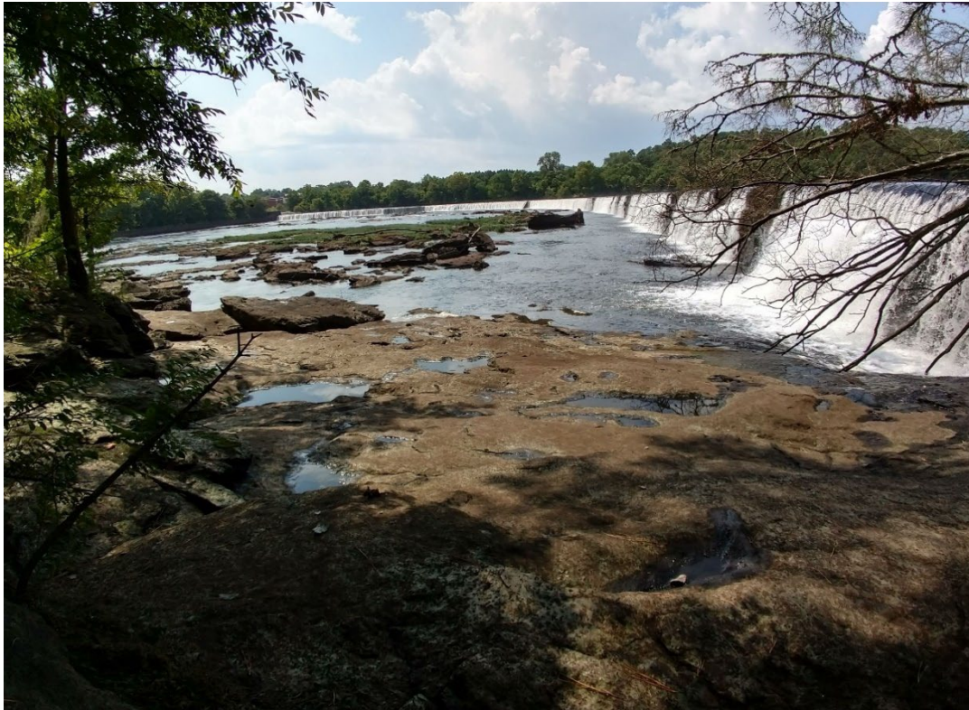
Note: View looking west from Georgia side of the Chattahoochee River at the Langdale Dam
