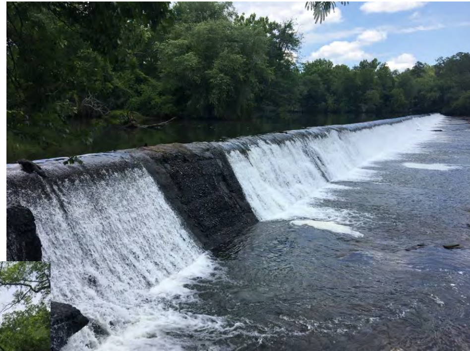
Crow Hop Dam
