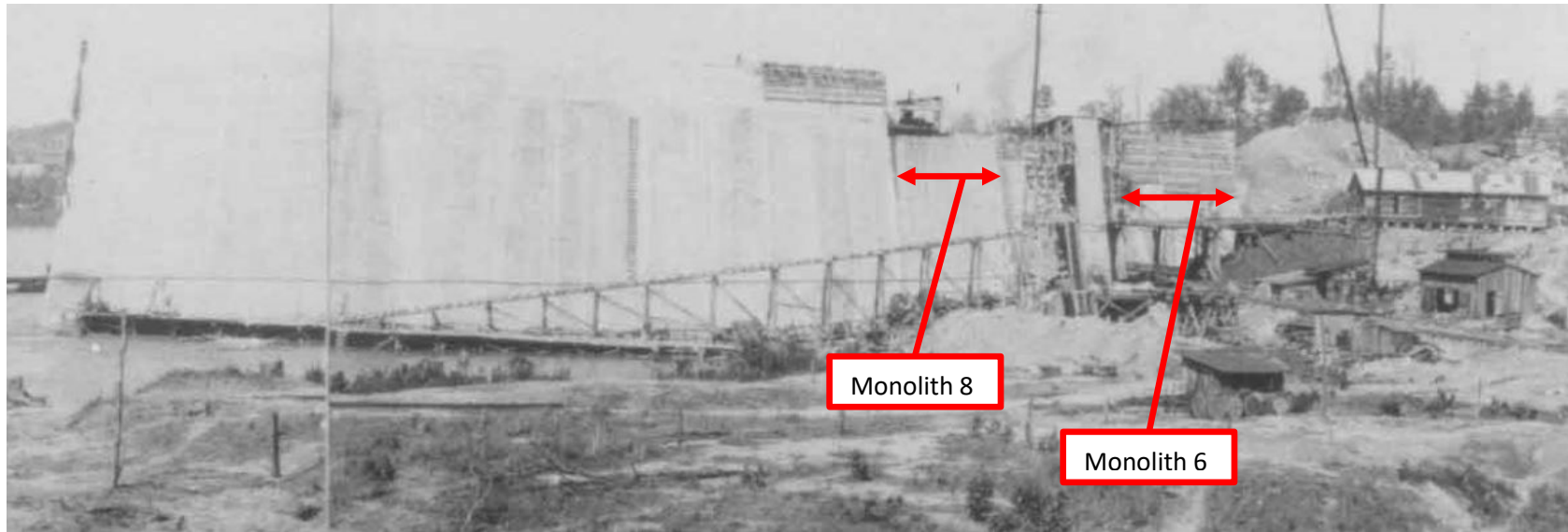
Figure 124. Spillway Monoliths Construction Progress as of 4/17/1910
