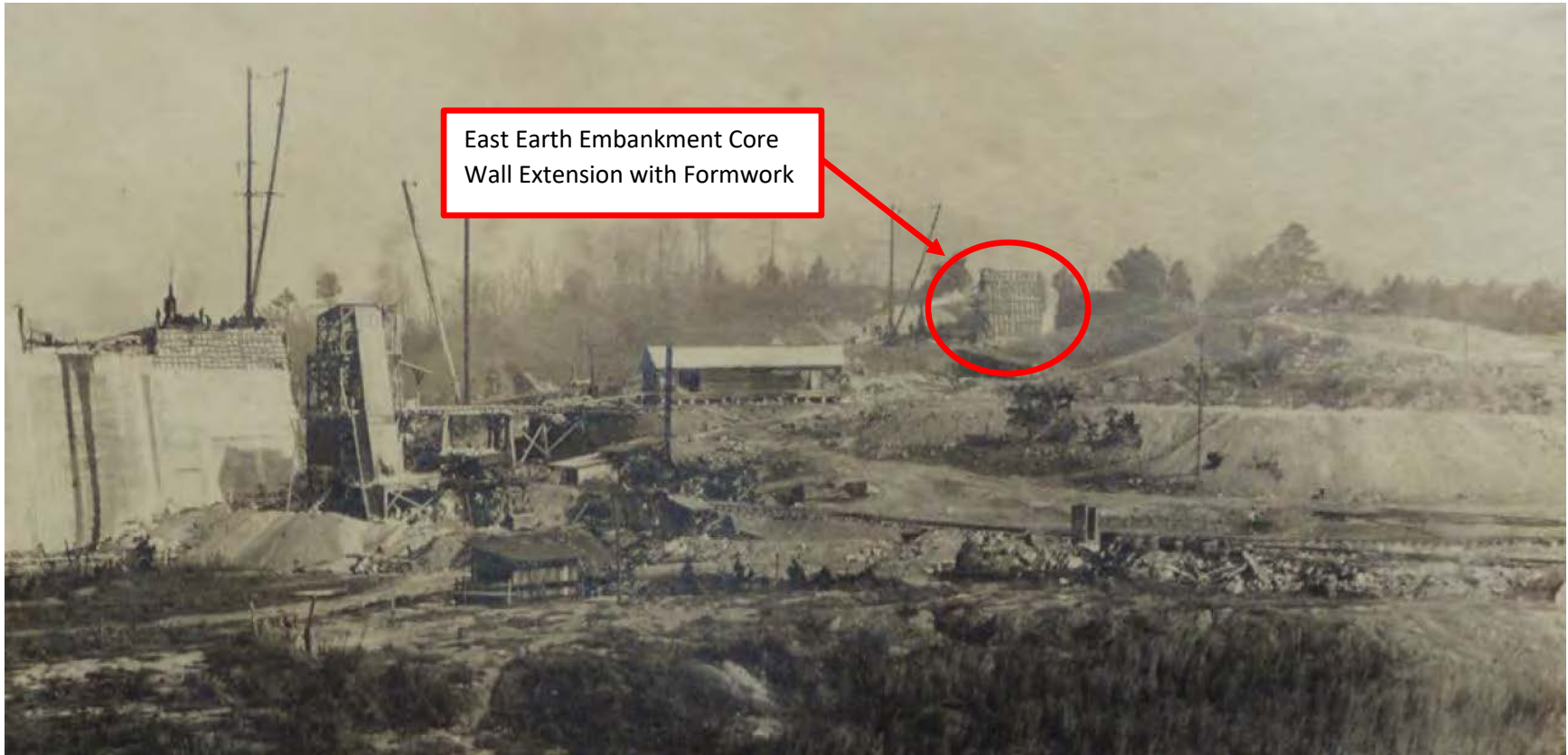
Figure 100. East Earth Embankment Core Wall as of 12/31/1909
