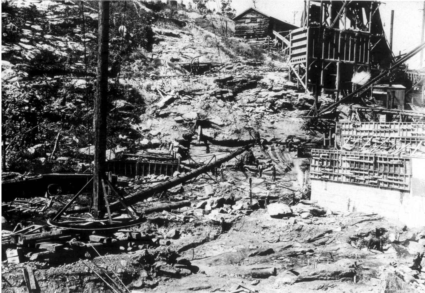
Figure 81. West Abutment Excavation
