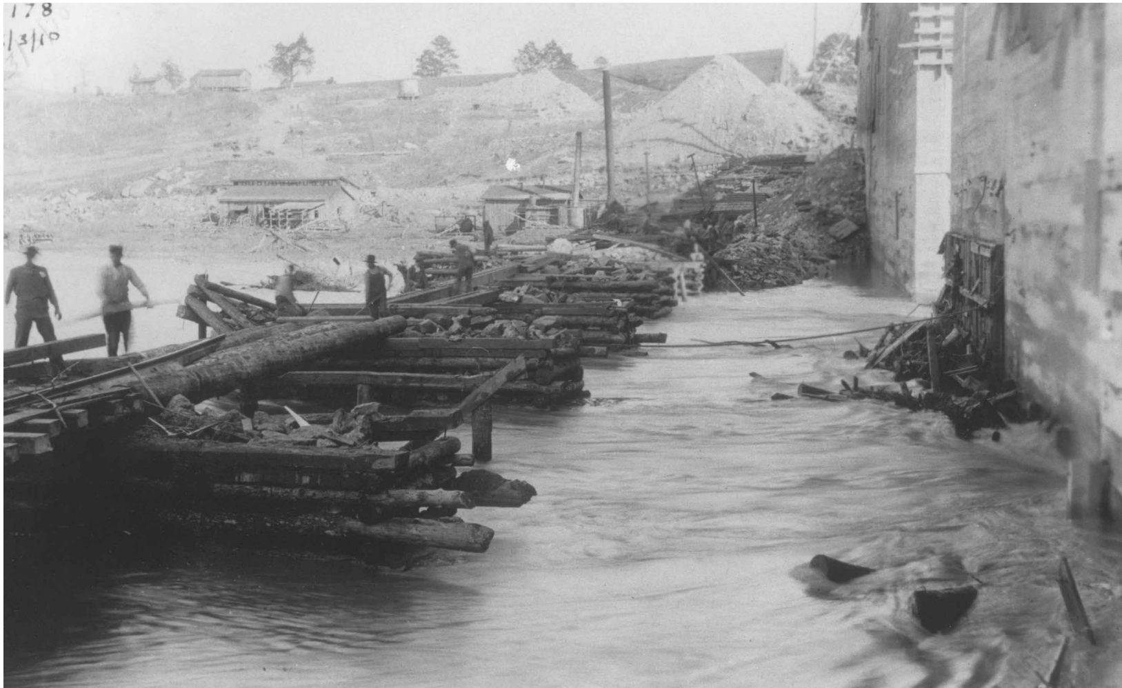
Figure 113. Upstream Original Construction Bridge Demolition
