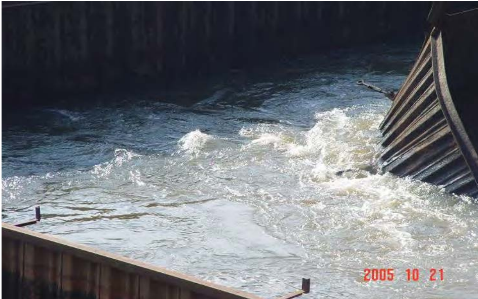
Figure 217. Weir Failure
