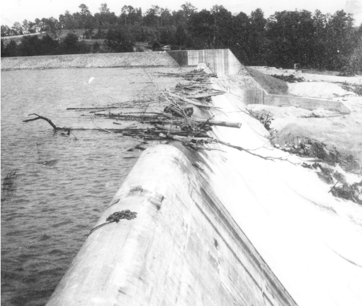
Figure 195. Spillway Crest and Debris
