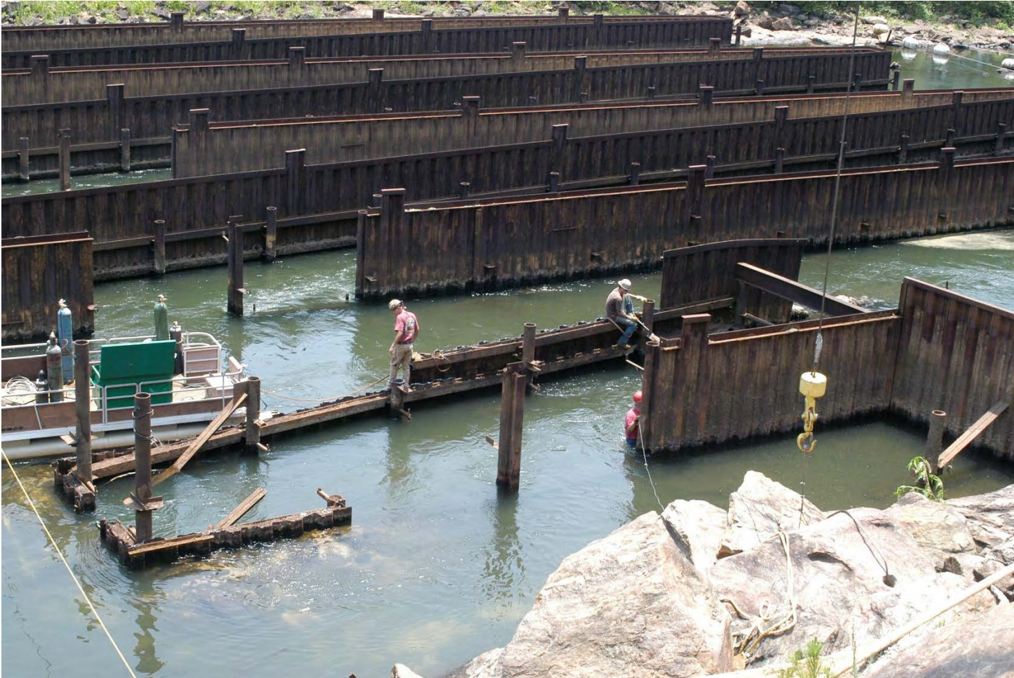
Figure 221. Weir Demolition as of 7/7/2008
