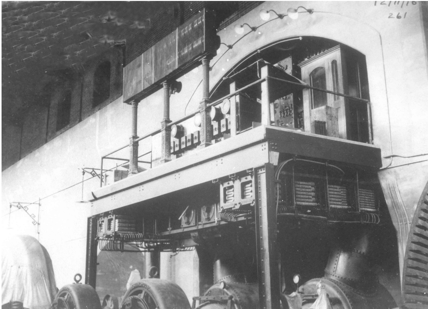
Figure 171. Operator's Platform as of 12/11/1910
