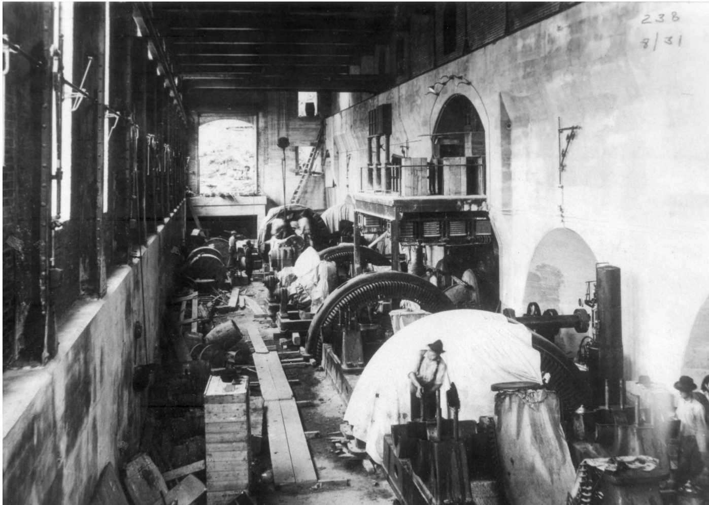
Figure 151. Powerhouse Generator Erection
