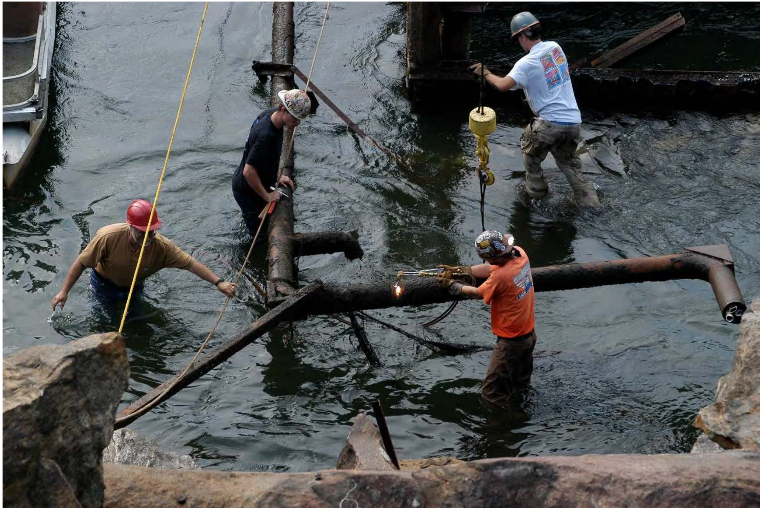
Figure 219. Monitor Piping Removal
