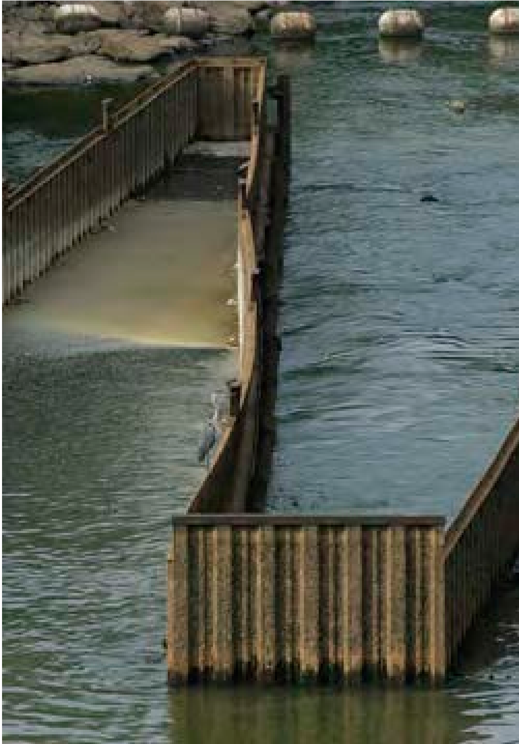
Figure 211. Weir Wall as of 8/10/2004
