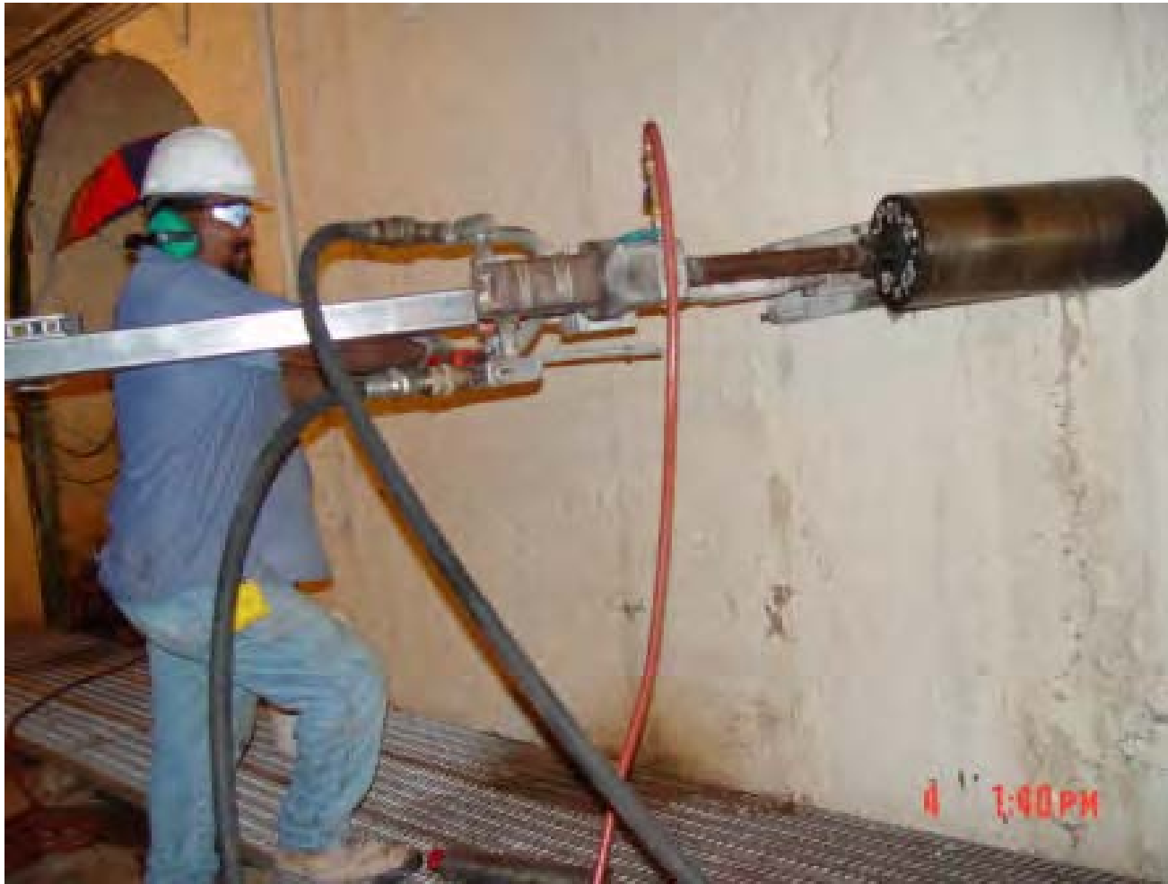
Figure 234. Coring Aeration Pipe Penetration
