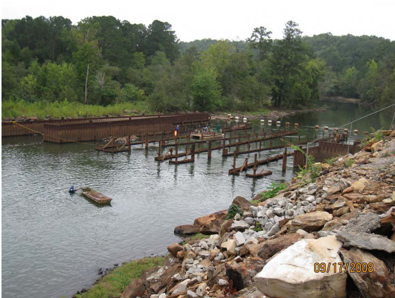
Figure 222. Weir Demolition as of 9/17/2008
