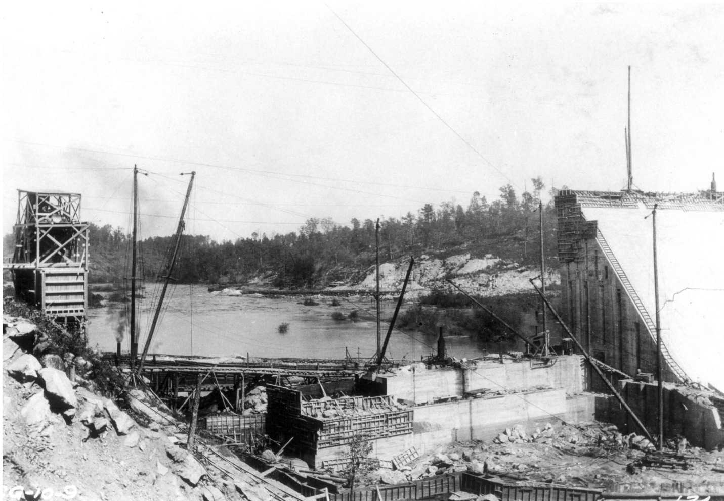
Figure 80. Intake/Powerhouse Construction Progress as of 10/9/1909
