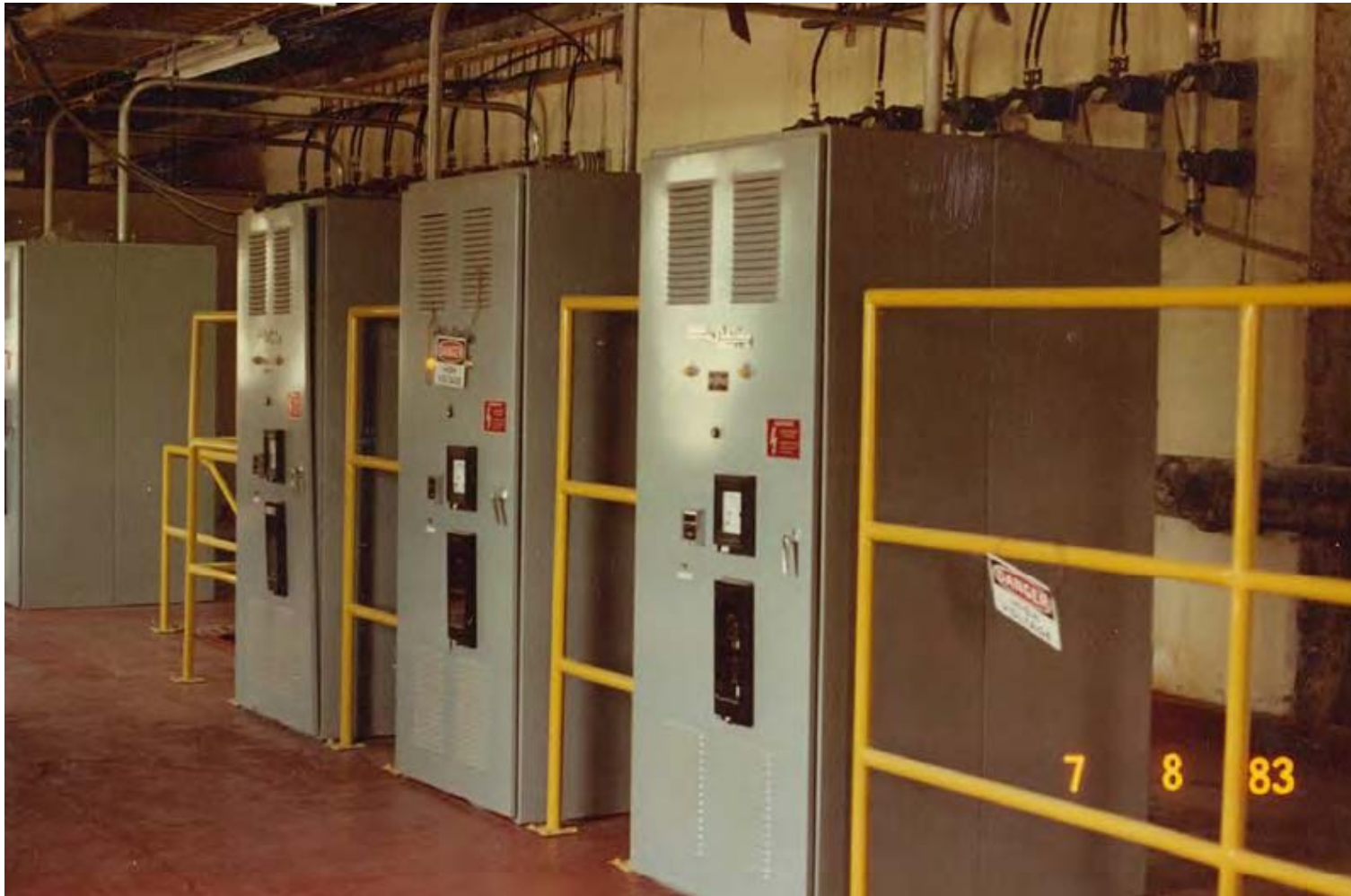
Figure 206. Solid State Exciters
