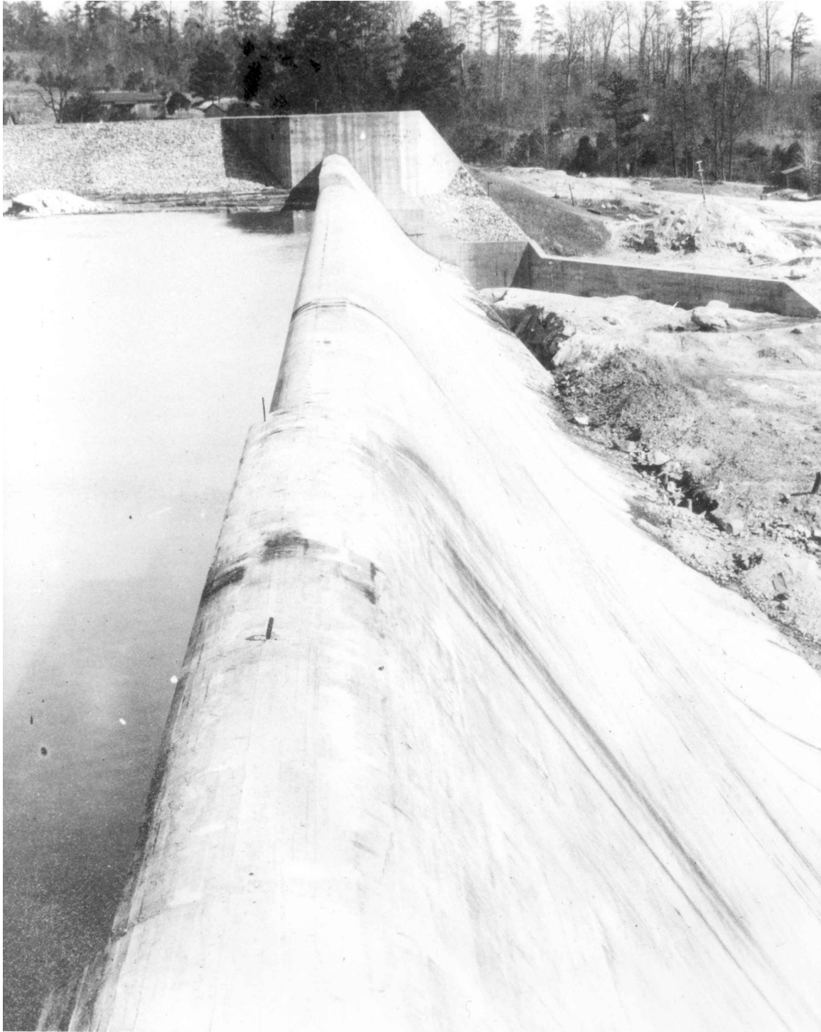
Figure 196. Completed Spillway Crest
