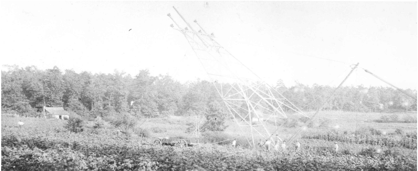
Figure 103. Transmission Line Tower Erection
