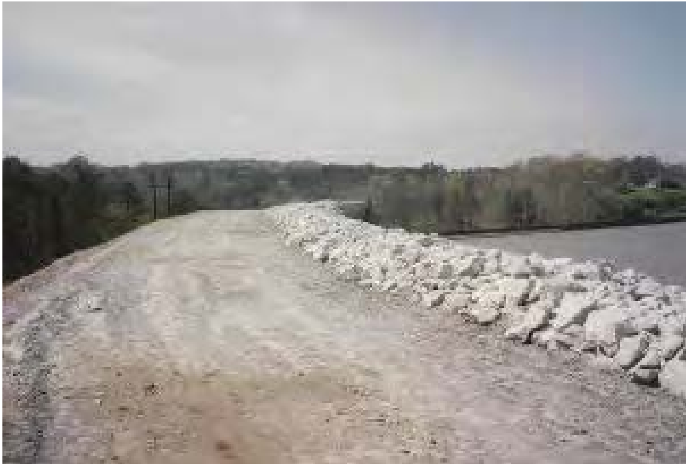
Figure 208. 1991 East Earth Embankment Modifications
