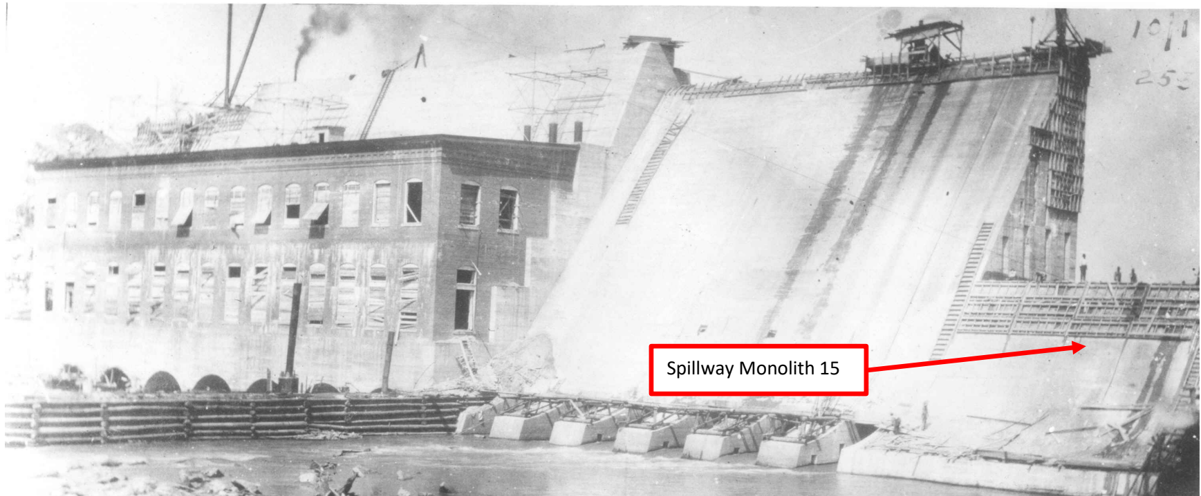
Figure 160. Spillway Monolith 15 Construction Progress as of 10/1/1910
