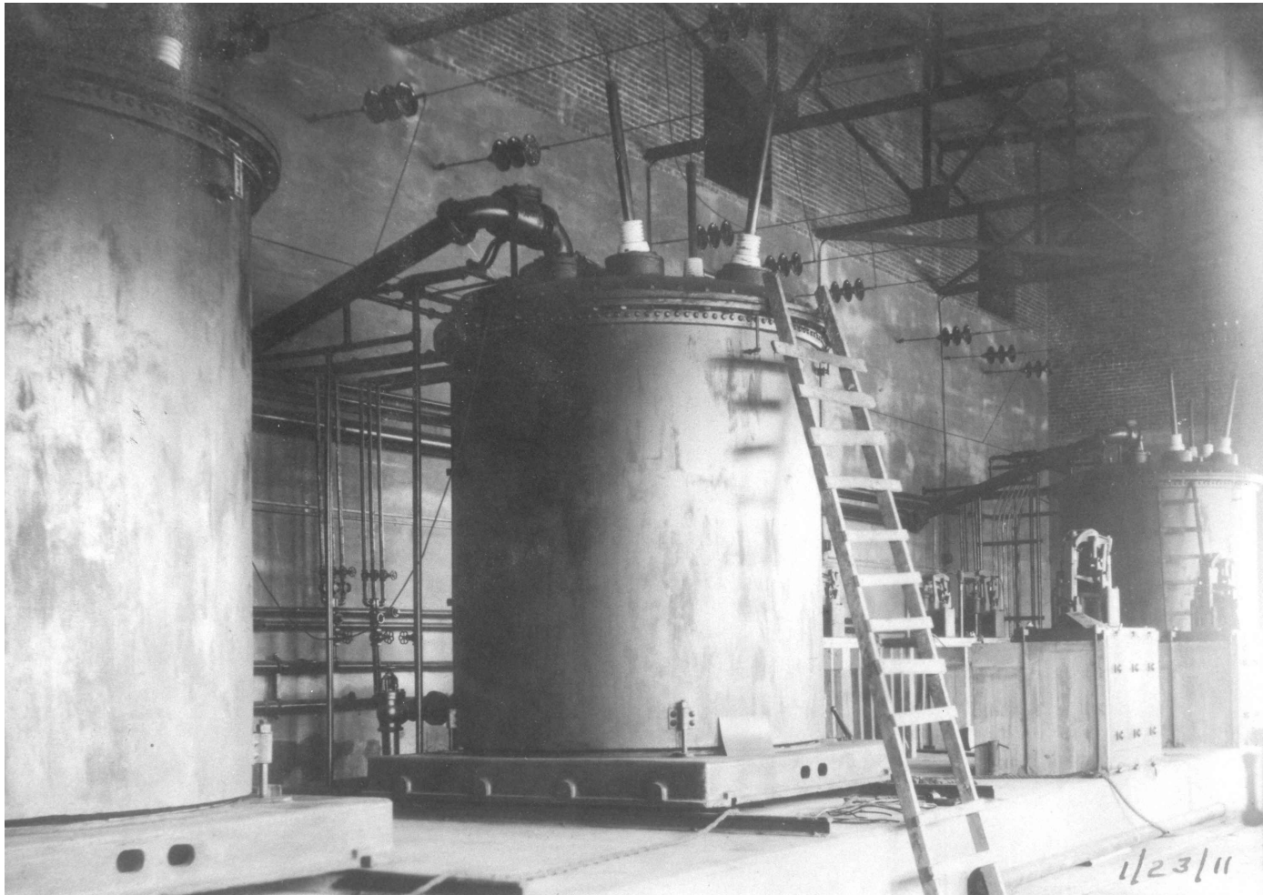
Figure 181. High-Tension-Floor 2,300/66,000 Volt Transformer, Piping, and Electrical Lines
