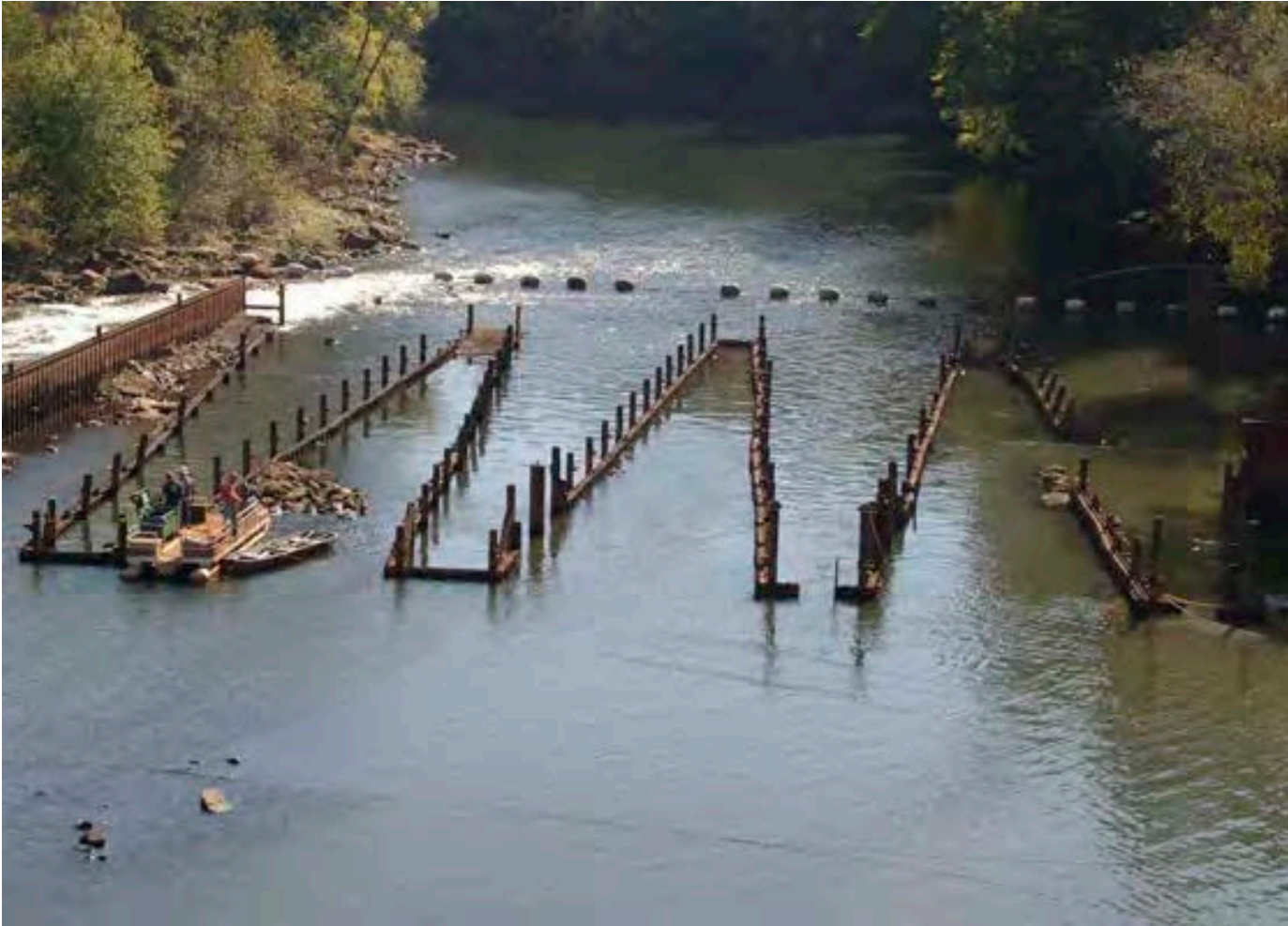
Figure 223. Weir Demolition as of 10/15/2008
