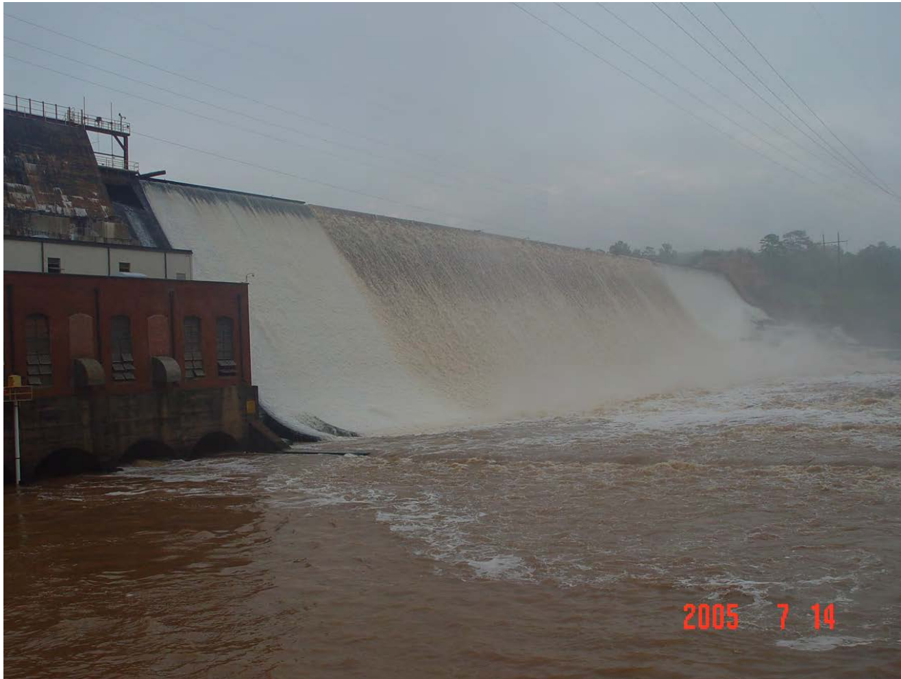
Figure 215. Spillway Discharges on 7/14/2005
