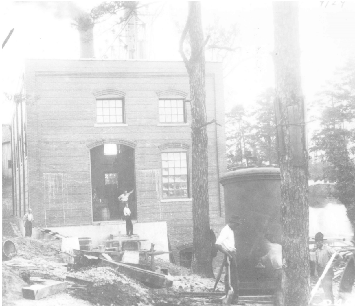
Figure 157. Substation Transformer Installation
