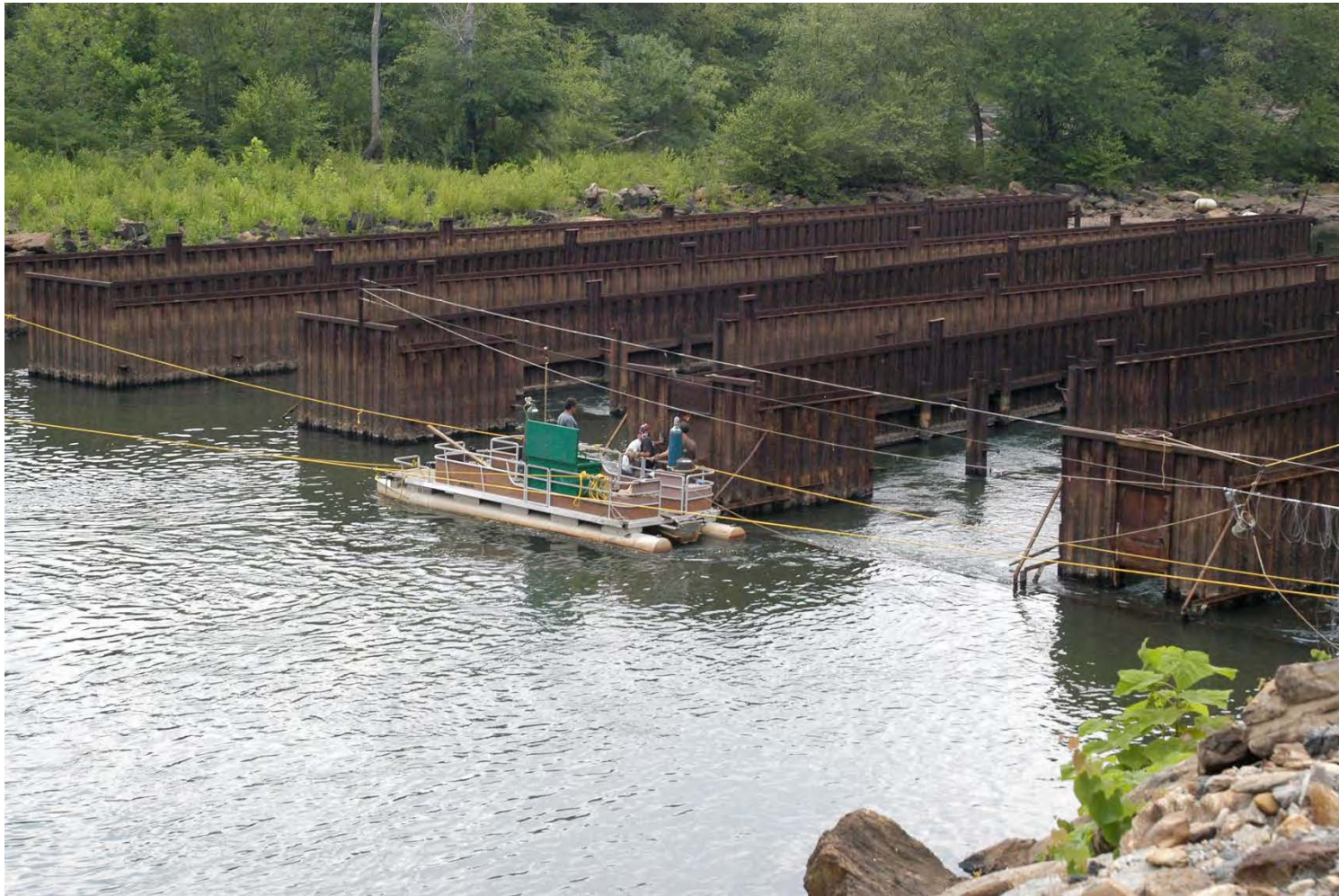
Figure 218. Weir Removal as of 6/26/2008
