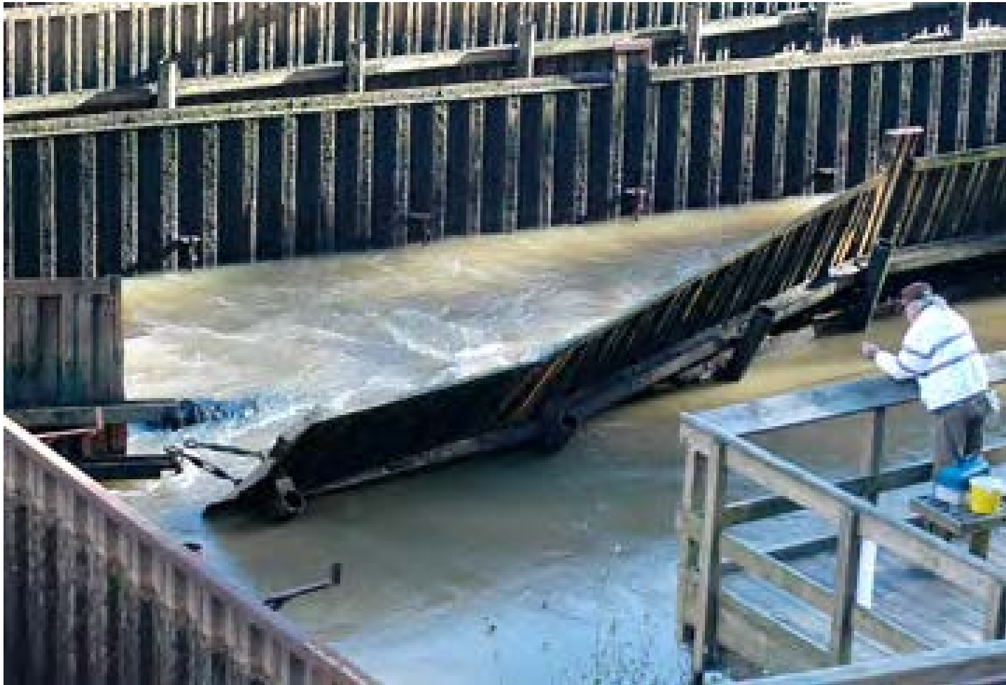
Figure 213. Separated Weir Wall
