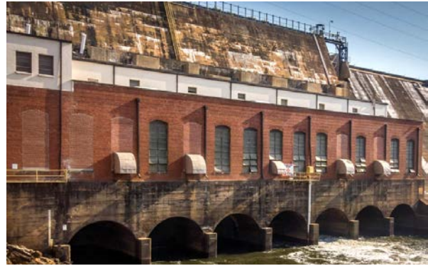
Powerhouse today, with upper floor half the size of the original
