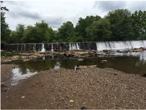
Photograph 3 - Crow Hop Dam.
