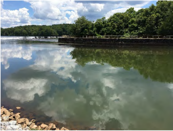
Photograph 1 - Area adjacent to dam.
