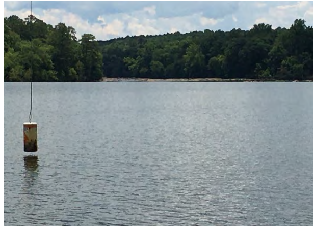
Photograph 2 - Shoals below dam.
