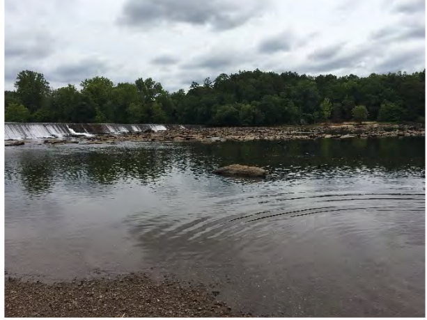
Photograph 2 - Eastern shoreline, downstream of dam.
