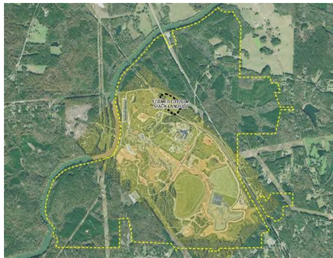
Plant Yates and the site
