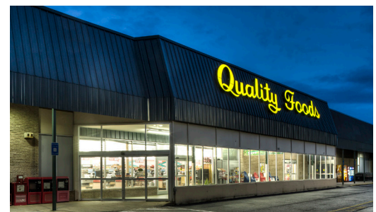
Quality Foods upgraded exterior canopy lighting and wallpacks to LEDs.
