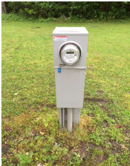
9.0 200 Amp, Customer Owned, UD Single-Phase Residential Socket
