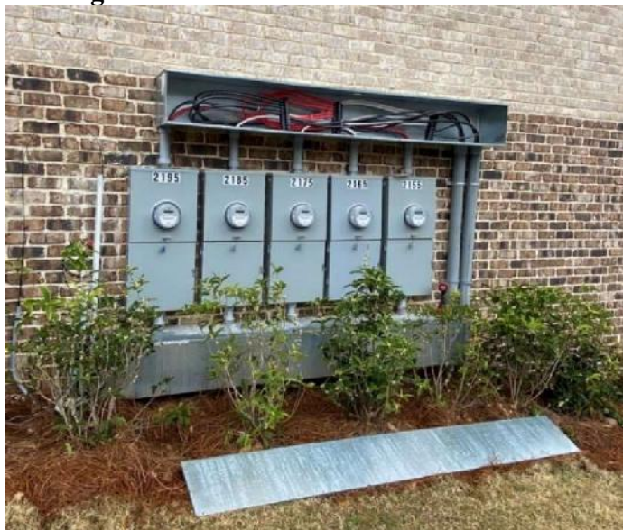
3.3 Single Phase Meter Socket & Auxiliary Gutter Installation
