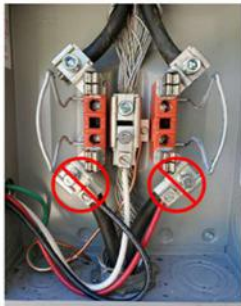
Modification to Factory Equipment including “accessory” chair lugs or hip clips
