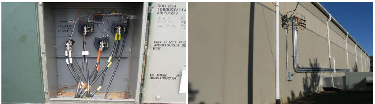
15.0 Pad Mount CT Installation and Wall Mount CT Installation
