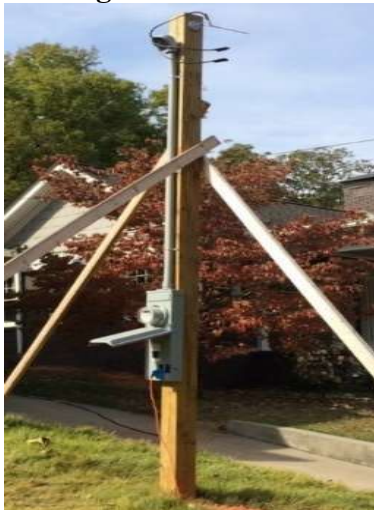
4.0 OH Temporary Service Installation
