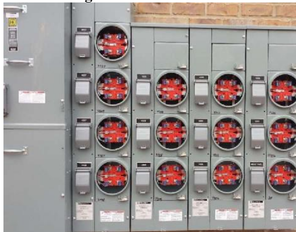
11.3 200 Amp, UD Multi-Gang Socket, Above 6 Positions
