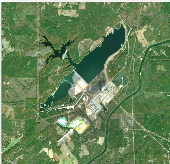
Plant Wansley and Plant Wansley Landfill
