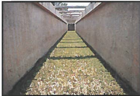
Channel Prepared for Testing
