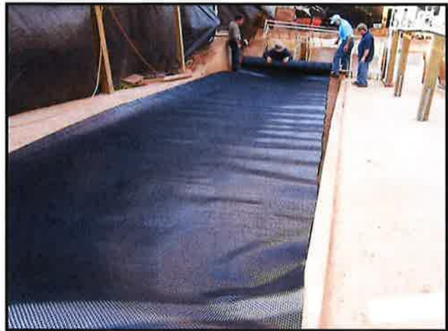
Test Slope Prepared and Liner Installed
