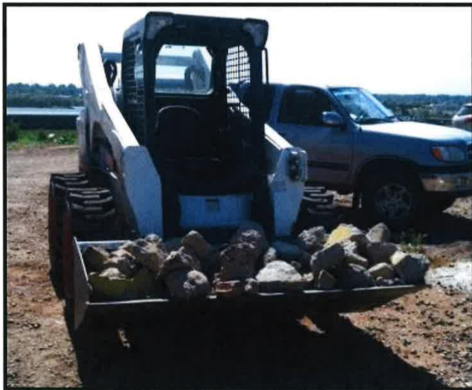
Figure 14 - Broken Concrete in Bobcat Bucket
