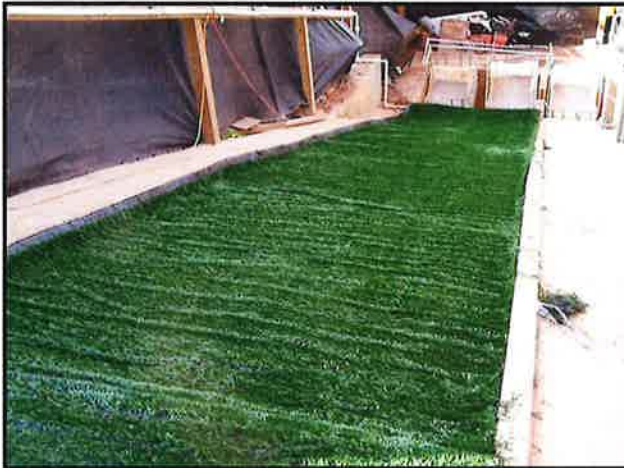
Synthetic Turf Deployed and Sand Ballast Layer Hand-Applied
