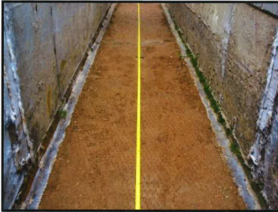
Figure 19 – Condition of the Soil Subgrade (After Testing and Removal of HydroTurf® System)
