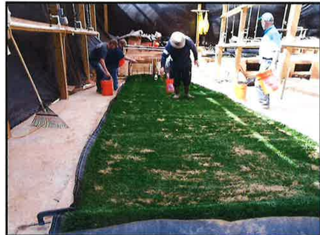
Synthetic Turf Deployed and Sand Ballast Layer Hand-Applied
