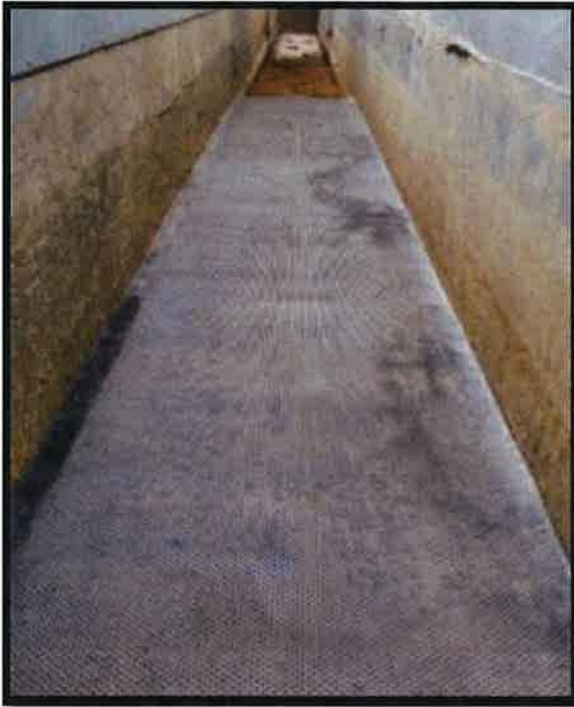
Figure 3 – Installation of the Structured Geomembrane
