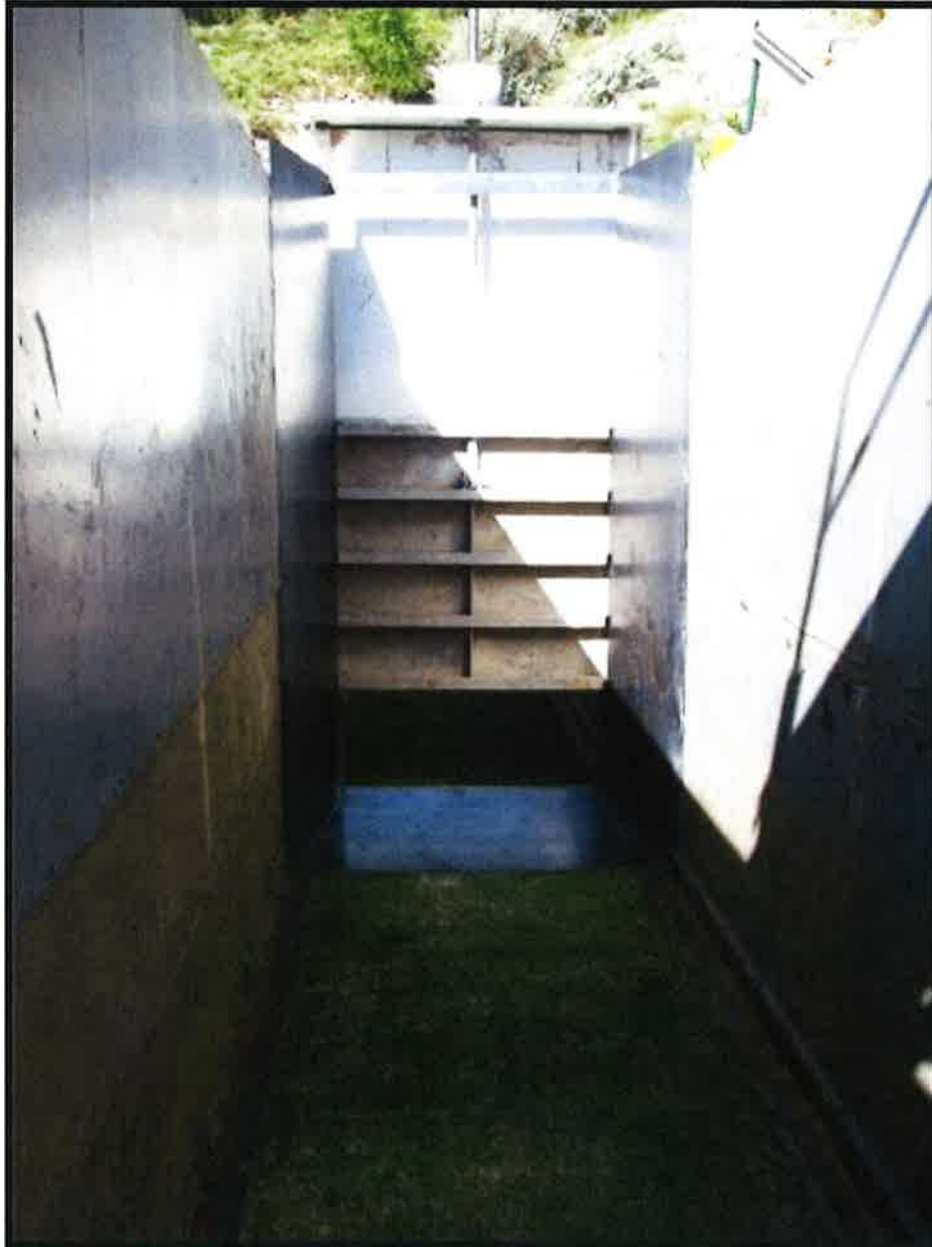
Figure 8 – Sluice Gate Installed in Overtop Flume for Hydraulic Jump Testing
