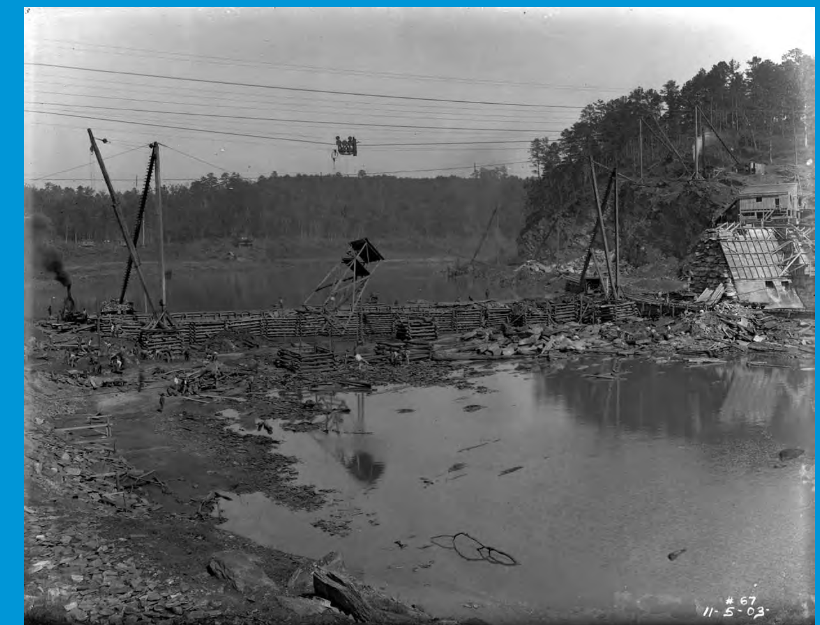
Towers and cables crossing the Chattahoochee River during construction.
