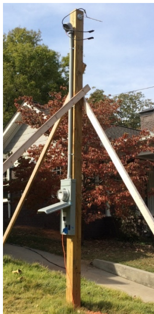
OH Temporary Service Installation
