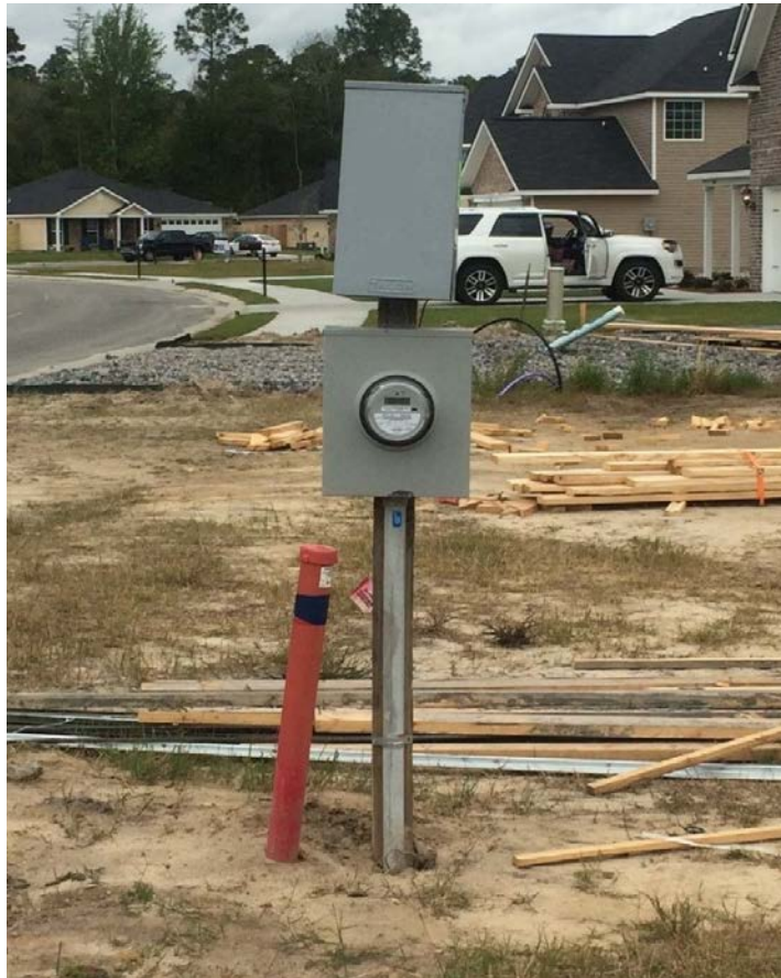
UD Temporary Service Installation
