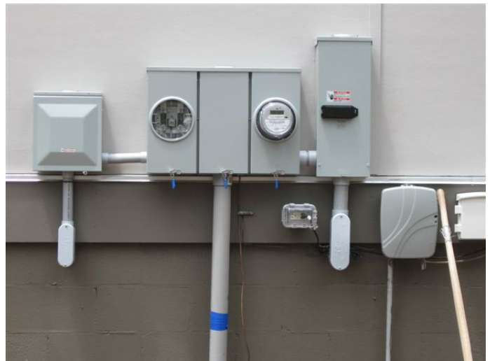
Residential (SP) 2 Meter Socket Configuration, Option 3
