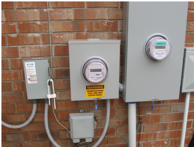
Residential (SP) 2 Meter Socket Configuration, Option 3
