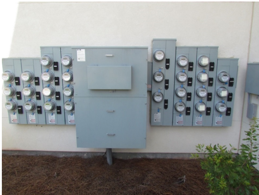
200 Amp, UD Multi-Gang Socket, Above 6 Positions
