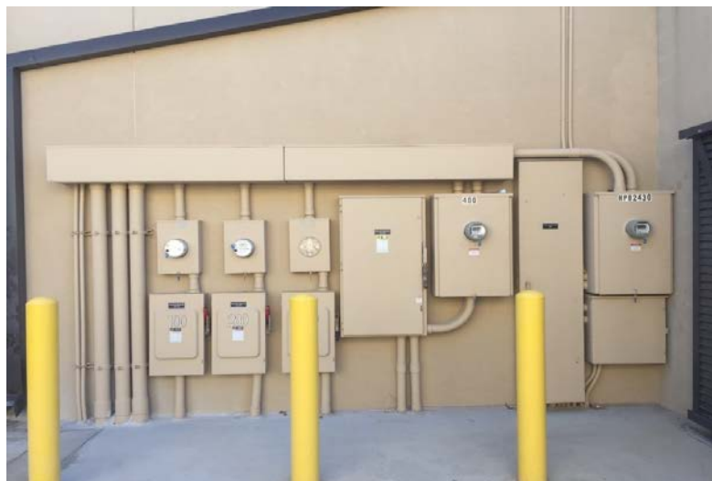
Typical Multi-Meter Distribution Point
