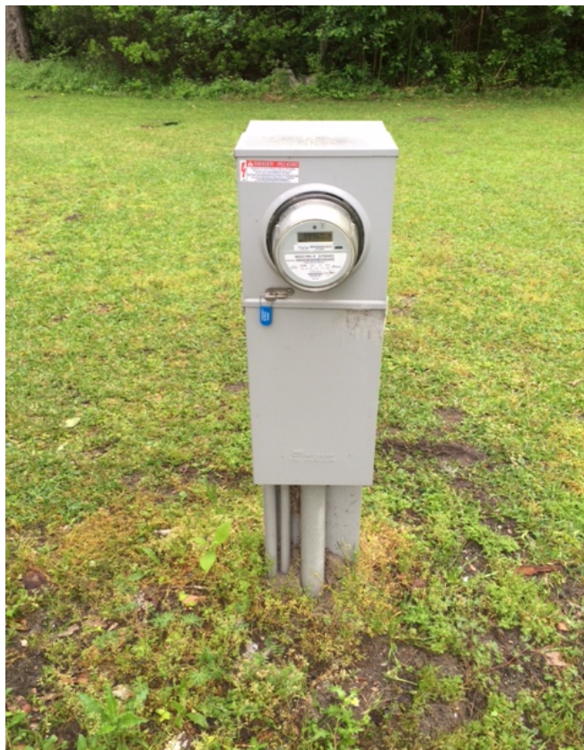
200 Amp, Customer Owned, UD Single-Phase Residential Socket
