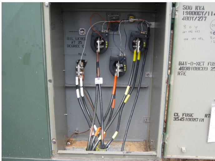
Pad Mount CT Installation and Wall Mount CT Installation
