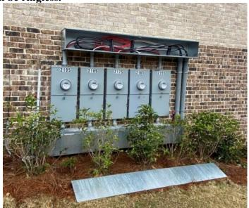
3.3 Single Phase Meter Socket & Auxiliary Gutter Installation
