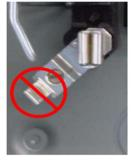
Socket lugs with factory "bypass horns"
