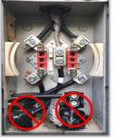
Wire taps, Utilco's, or other clamp-on wire piercing devices
