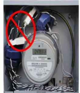
Customer owned CT meters and instrument transformers
