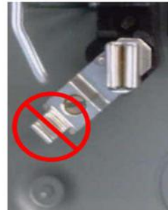
Socket lugs with factory “bypass horns”
