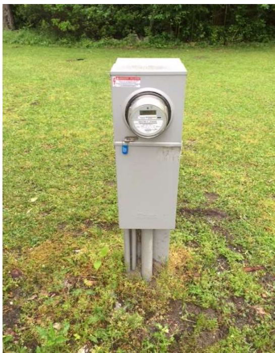
9.0 200 Amp, Customer Owned, UD Single-Phase Residential Socket
