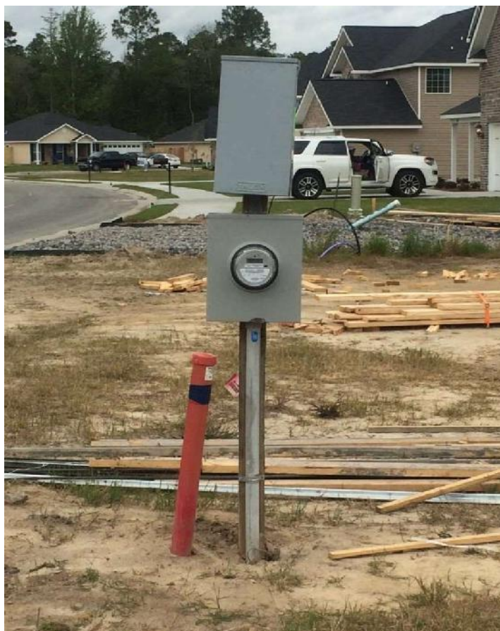
4.2 UD Temporary Service Installation
