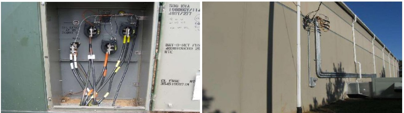
15.0 Pad Mount CT Installation and Wall Mount CT Installation
