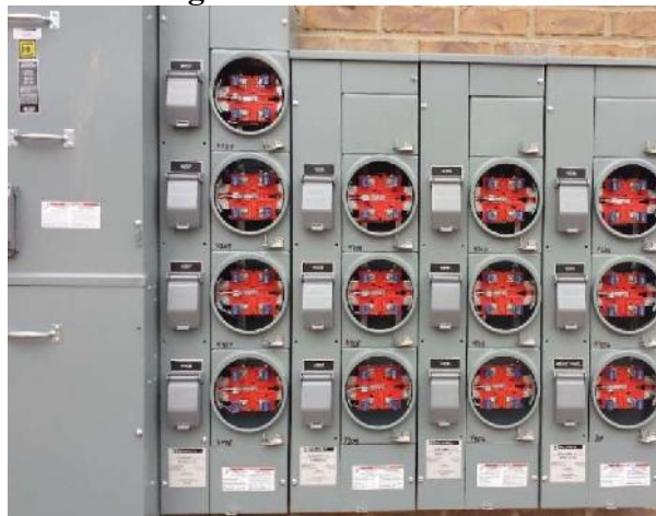
11.3 200 Amp, UD Multi-Gang Socket, Above 6 Positions
