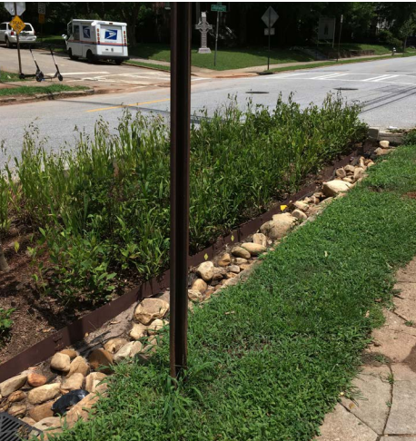
Residential stormwater planer installed by Trees Atlanta
