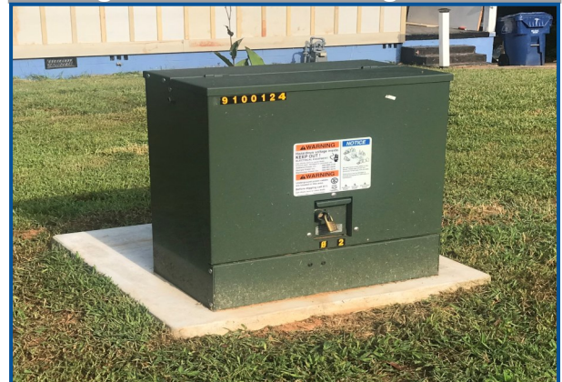
Single Phase Terminating Cabinet
