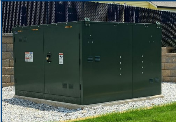
Switching Cubicle
