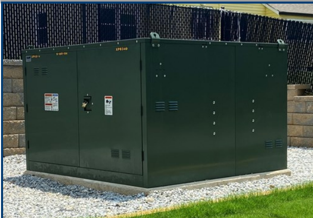
Switching Cubicle
