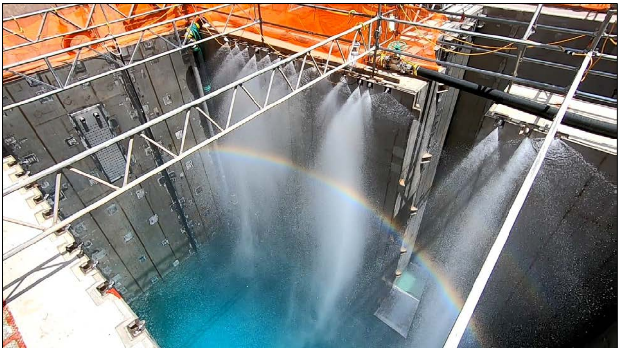
Unit 3 Spent Fuel Pool Cooling System spray header flush
