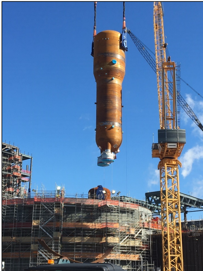
Steam Generator being set inside Unit 4 Containment
