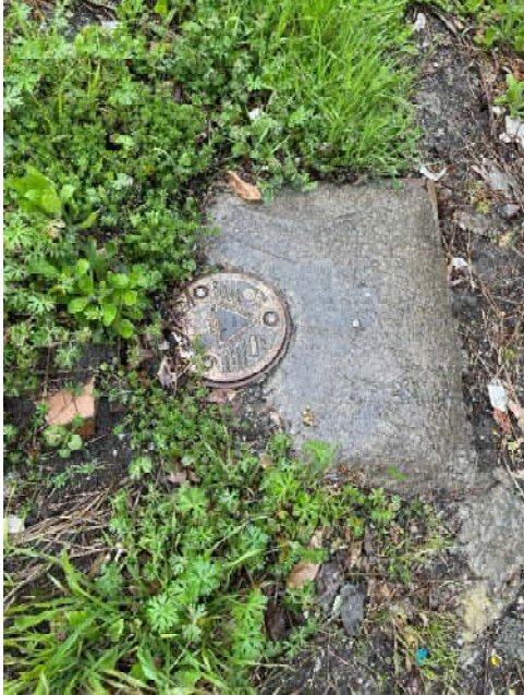
B-97 – Installed locking bar.
