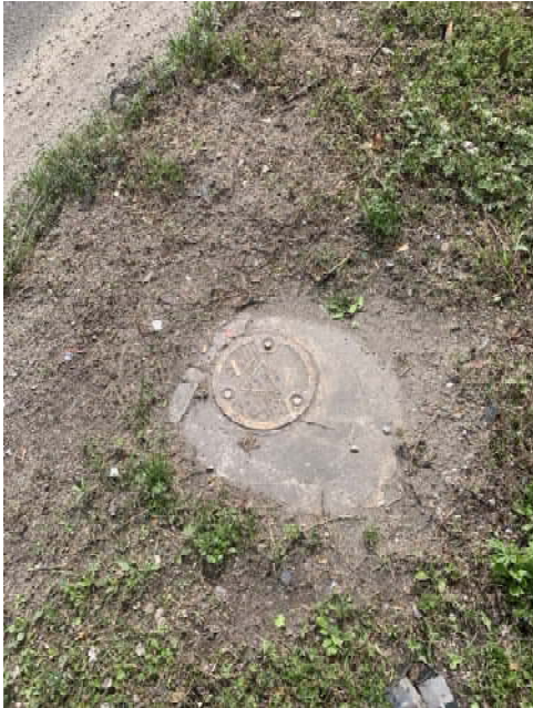
B-96 – Installed Locking bar.
