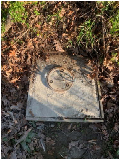
B-98 – Installed locking bar.
