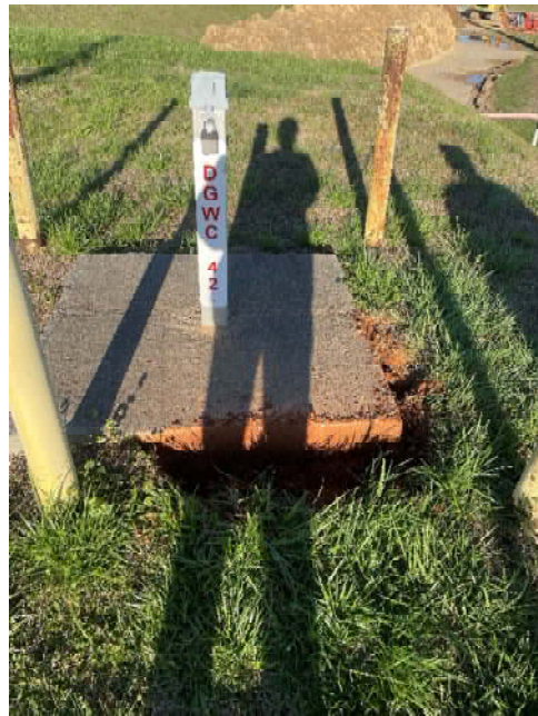
B-62 – Reinstalled bolts. (Notes indicated broken bracket. After inspection bracket was not broken, bolts laying inside the cover.)
