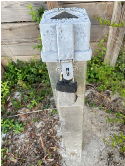
B-94 – replaced well cap so the protective cover will lock.
