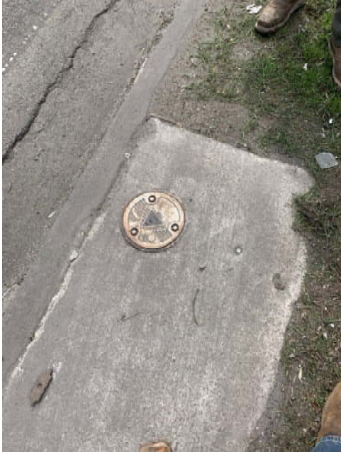
B-95 – Installed locking bar.
