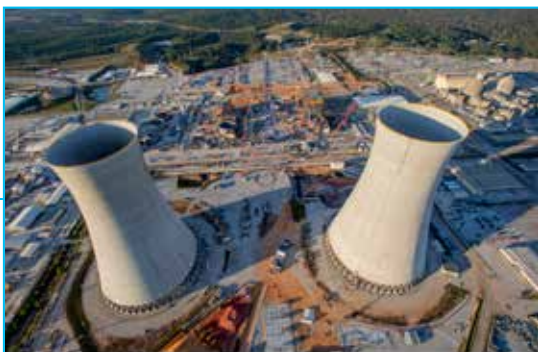
New units at Plant Vogtle
