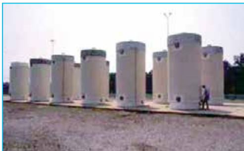
Plant Vogtle began loading the first of its used fuel into casks in 2013.
