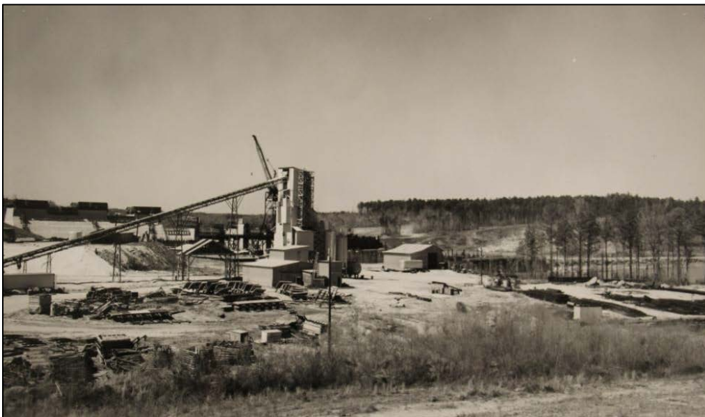
Figure 11. The Concrete Batch Plant, View North (Source: Wallace Dam Photograph Archives)
