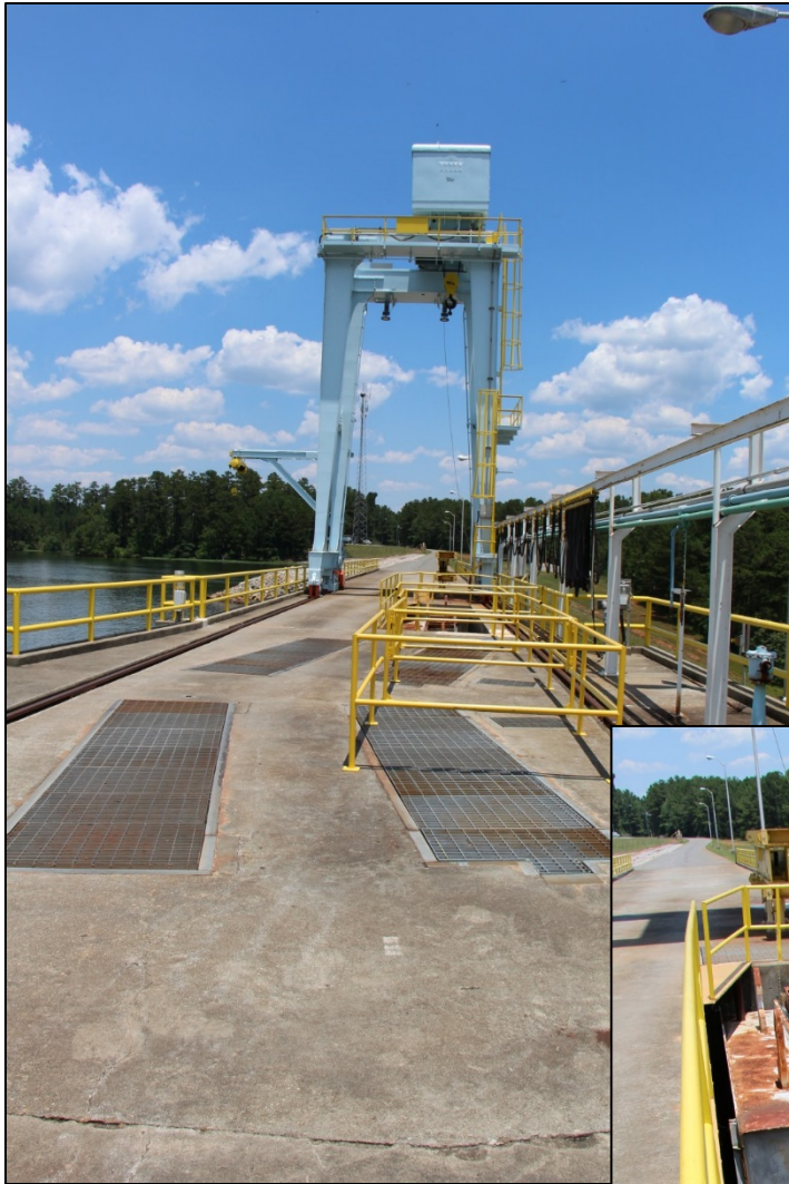
Figure 32. View East Across Top of Dam Headworks Toward Gantry Crane that Controls Stop Logs, View Northeast
