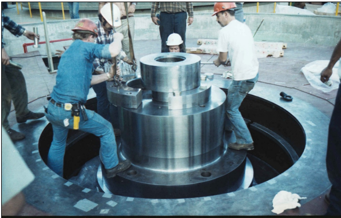
Figure 24. Workers Installing a Generating Unit at Wallace Dam, 1979 (Source: Georgia Power Company Archives)
