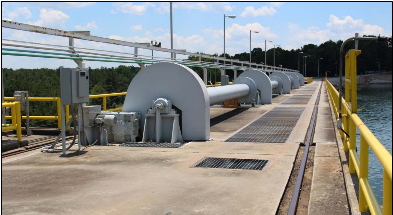
Figure 35. Spillway Tainter Gate Hoists, View Southwest
