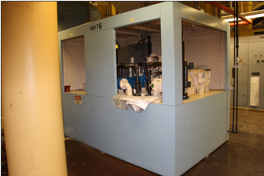
Figure 40. Unit 6 Governor Cabinet Controls the Position of the Turbine Wicket Gates
