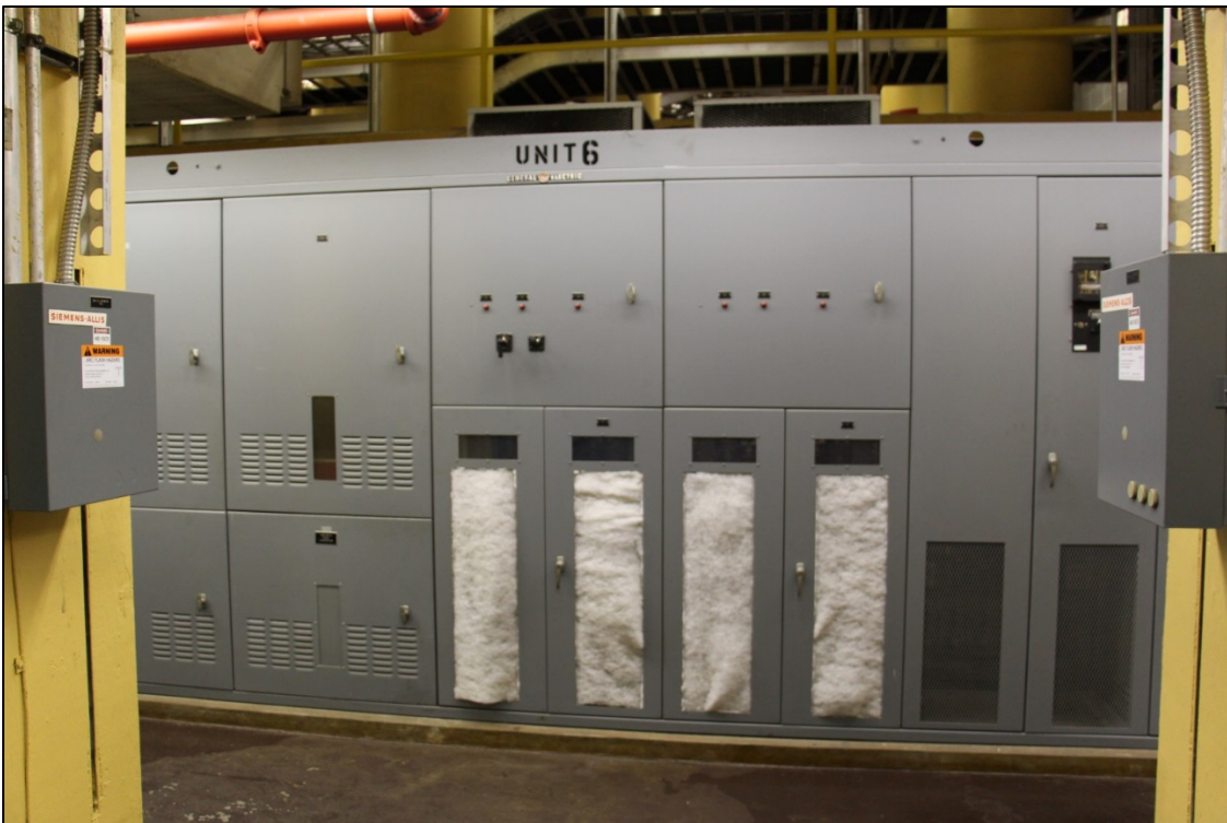
Figure 41. The Unit 6 Exciter Cabinet Generates the Magnetic Field in the Generator
