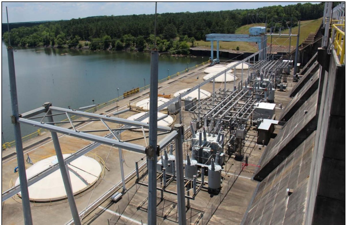
Figure 31. View of the Powerhouse Deck From Above Showing Generating Unit Covers, Gantry Crane, and Substation, View Southwest
