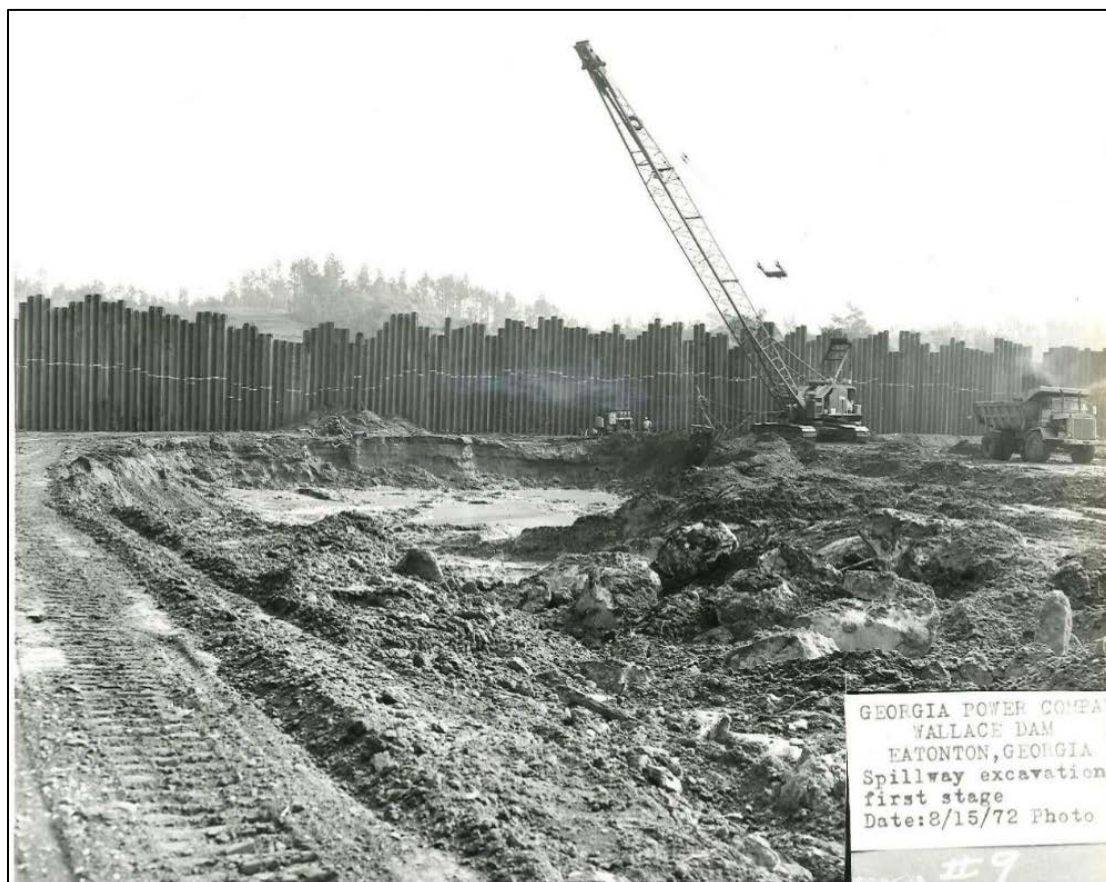
Figure 12. First Stage Diversion Cofferdam and Rock Excavation for Spillway, View East, August 15, 1972 (Source: Southern Company Hydro Services: 238)
