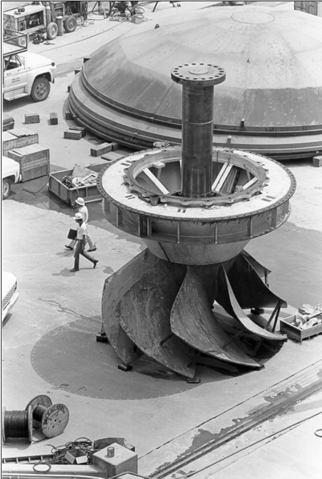
Figure 21. Turbine Runner Readied for Installation at Wallace Dam, 1979 (Source: Georgia Power Company Archives)
