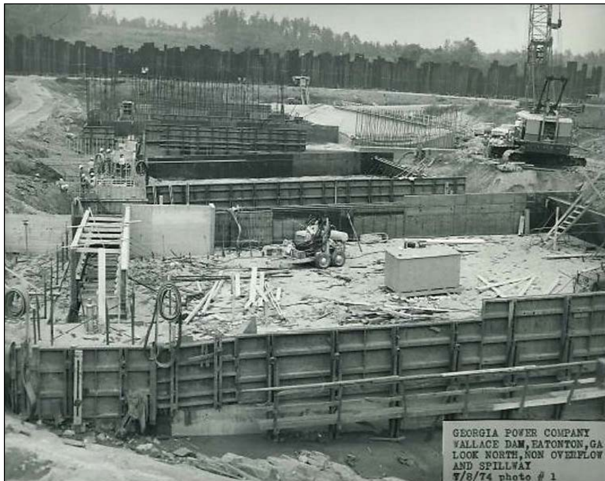
Figure 15. Construction of the West Nonoverflow and Spillway Foundations, July 8, 1974 (Source: Southern Company Hydro Services: 244)
