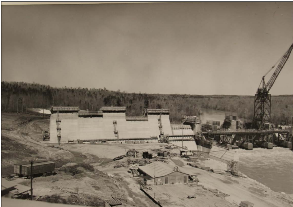
Figure 17. West Nonoverflow Section and Spillway Piers during Second Stage of Construction, March 26, 1975, View Northwest From Concrete Batch Plant (Source: Wallace Dam Photo Archives)
