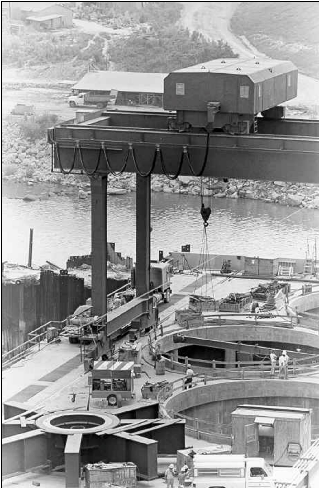
Figure 22. Bridge Crane Installing Turbine and Generator Components, 1979 (Source: Georgia Power Company Archives)
